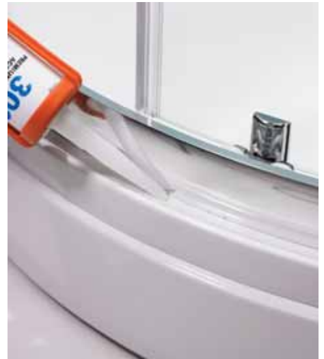
18 Push fit the tray skirt and seal around the front of the enclosure using silicone.
