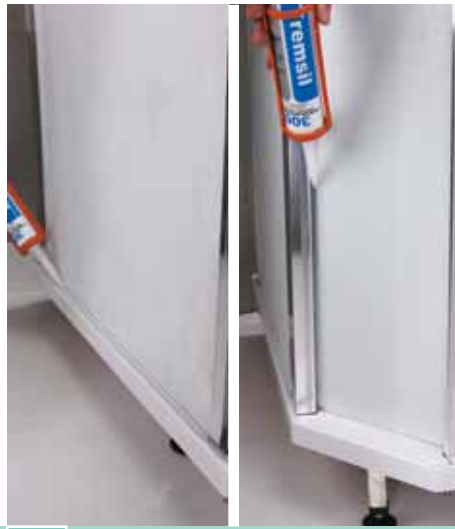
14 On the rear of the unit, silicone between the tray and glass panels. Also silicone from the base up 150mm, where the panels interlock.
