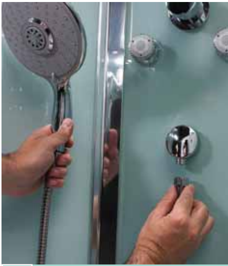
13 Attach the shower hose and position the shower head.
