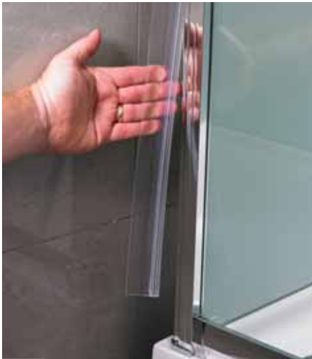
16 Push fit the wall seals on either side of the unit.
