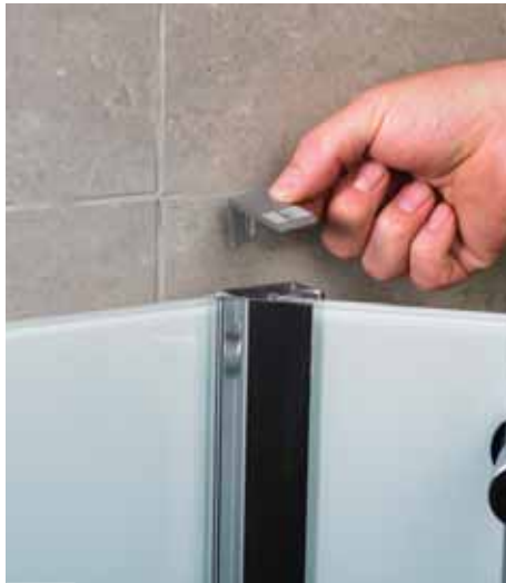
17 Mark up and fix the wall bracket to secure the unit to the wall.
